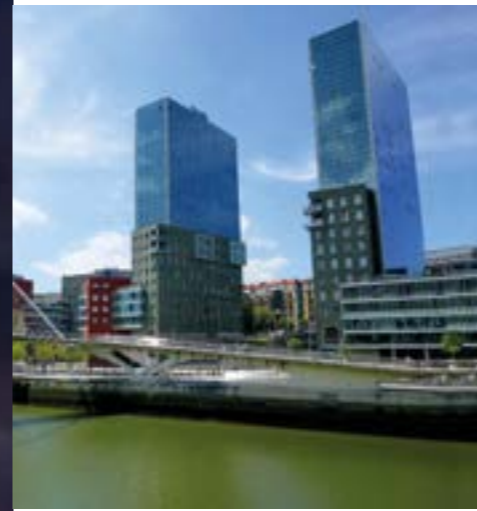
Isozaki Towers. SPAIN
